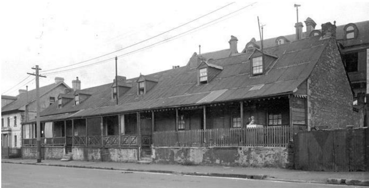
107-111 Princes St, 1926 (No 107, the Chester residence is probably on the right)
