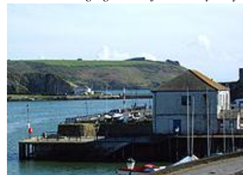
Phoenix Wharf – The only remaining building associated with Plymouth Emigration Depot
